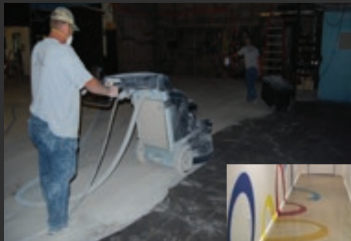
COATING REMOVAL & FLOOR PREP
